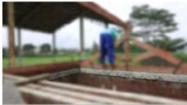
Gambar II.381 Balok Keliling/ ring
