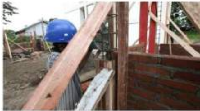
Gambar II.415 Proses Pengecoran Kolom
